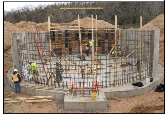
Pictured is one of the two 50 foot diameter primary clarifiers being constructed. The purpose of the primary clarifiers is to separate solid particles in the wastewater mixture from the liquid.
